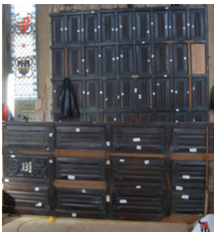
Repaired 16th-century panelling with new panel in background, and (below) the back of the panelling showing its repair.
