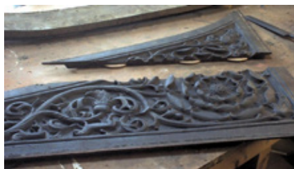
The use of unglued wooden biscuits to hold a two-piece spandrel panel in line while allowing movement
