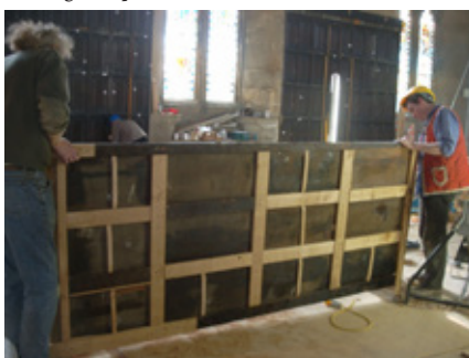
Repaired 16th-century panelling with new panel in background, and (below) the back of the panelling showing its repair.
